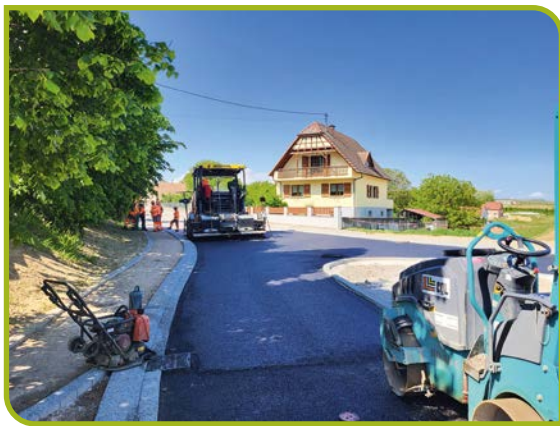
POSE GRAVE BITUME
